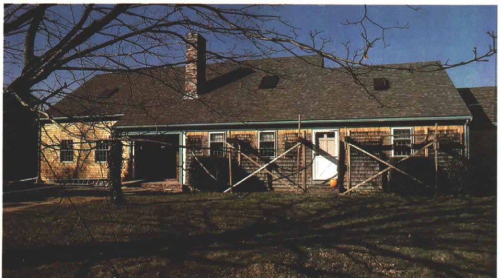
The finished house, seen from the front, appears smaller than it actually is because the extended roofline obscures the new 40-ft. shed dormer at the back of the house.
